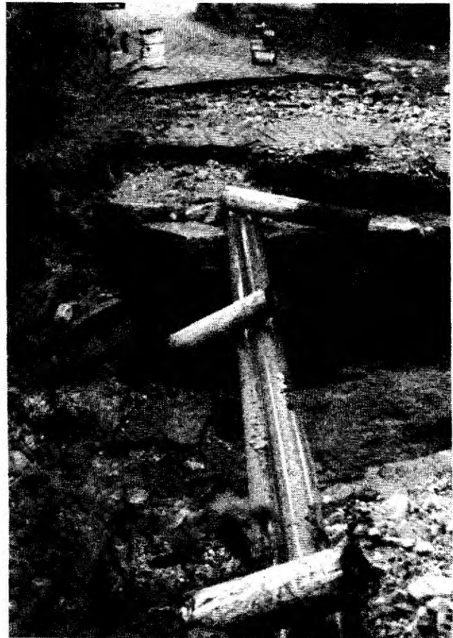
Reservoir Road Washout
