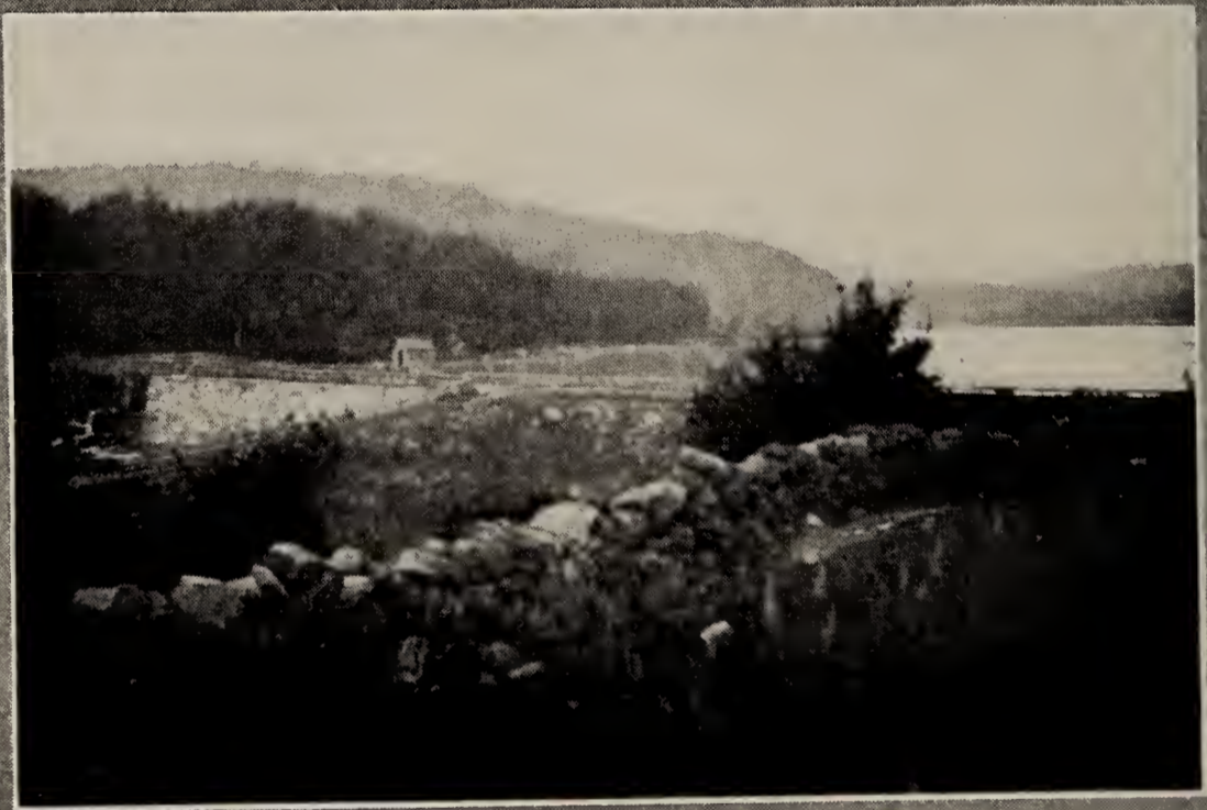
MAIN RESERVOIR—LOOKING EAST
