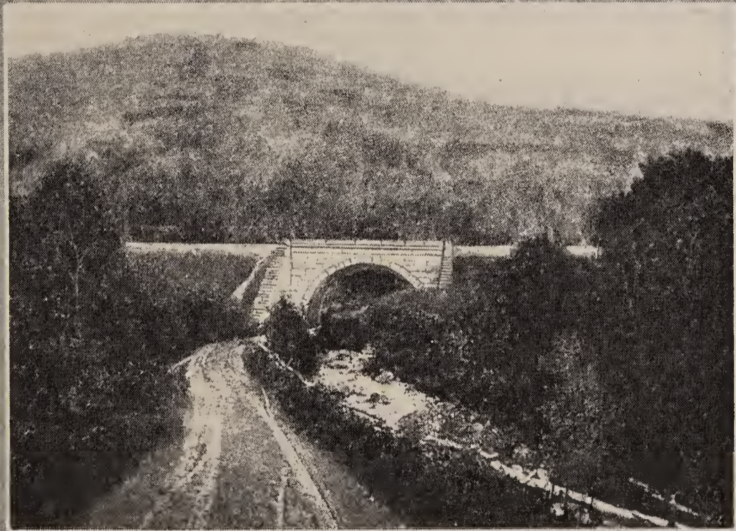
ROAD TO BANCROFT RAILROAD ARCH OVER FACTORY BROOK
