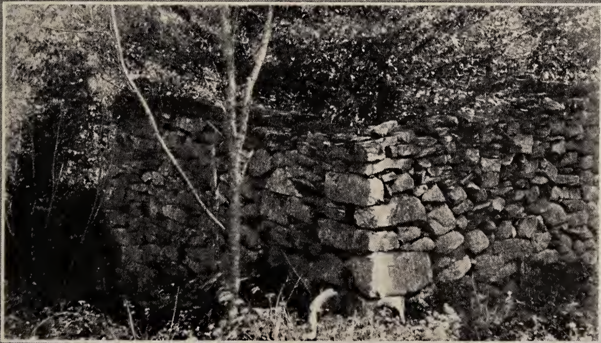
GLENDALE FALLS FOUNDATIONS OF RHOADS' MILL
